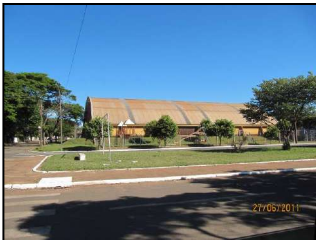
Figura 223 – Ginásio Municipal de Paranacity.
